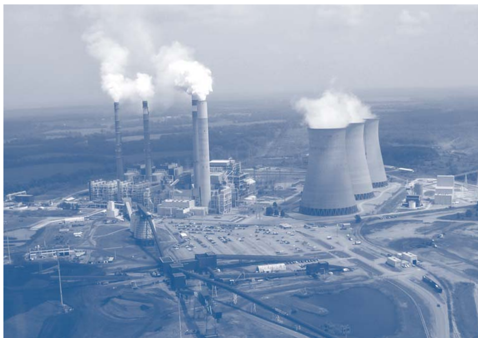
Paradise Coal-fired Plant, Western Kentucky
